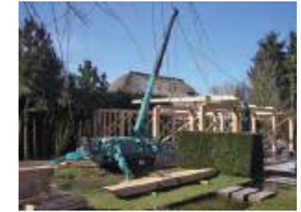
MC305C House Construction
