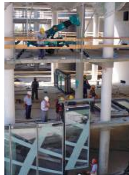
MC285C Construction Glass Lifting Bucharest
