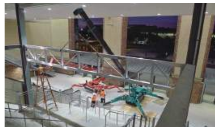
MC405C Steel Erection Kyle Field
