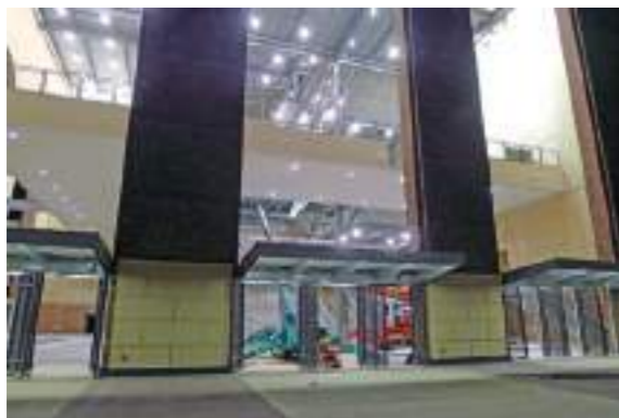
MC405C Sign Install - Inside Football Stadium US
