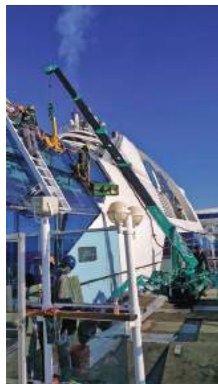
MC285C Ship Glazing On Upper Deck Of Cruise Ship US
