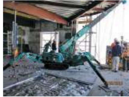
MC285C Construction Dubai Princess Tower
