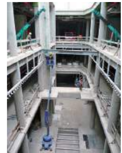
MC285C Construction Sky Tower
