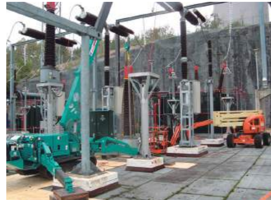
MC405C Power Station US
