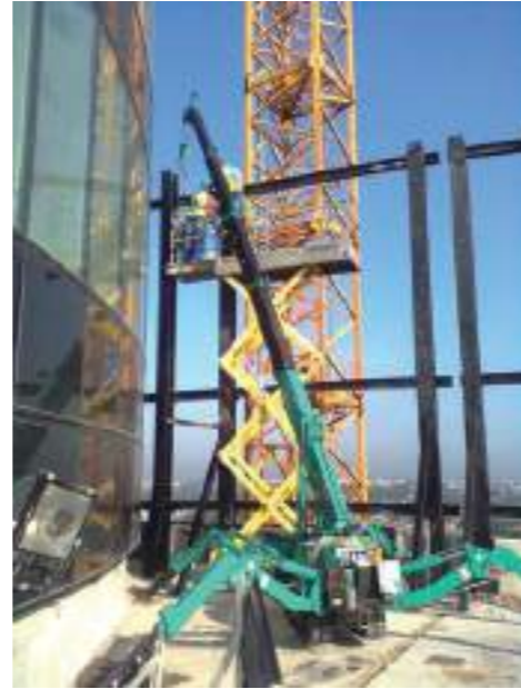
MC285C Rooftop Work
