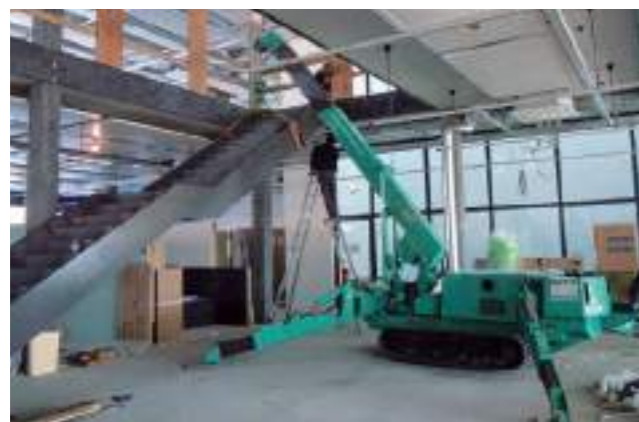
MC305C Construction Indoor
