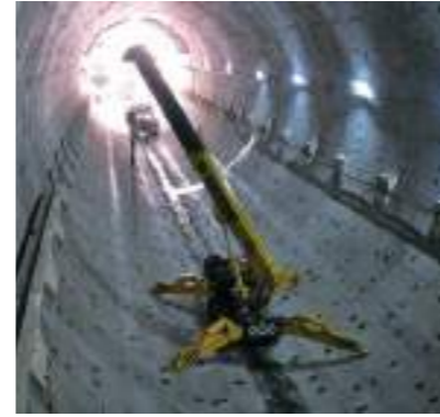
MC405C Tunnel Australia
