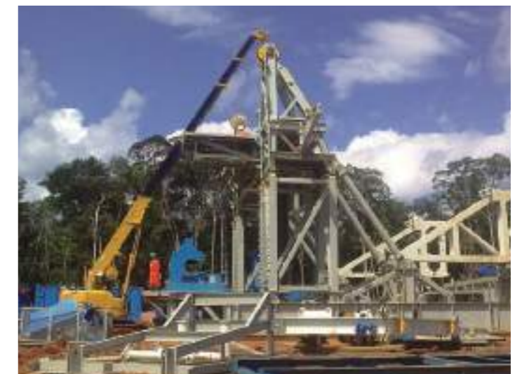
LC1385 On Site Rig Up of QG 5 Brazil
