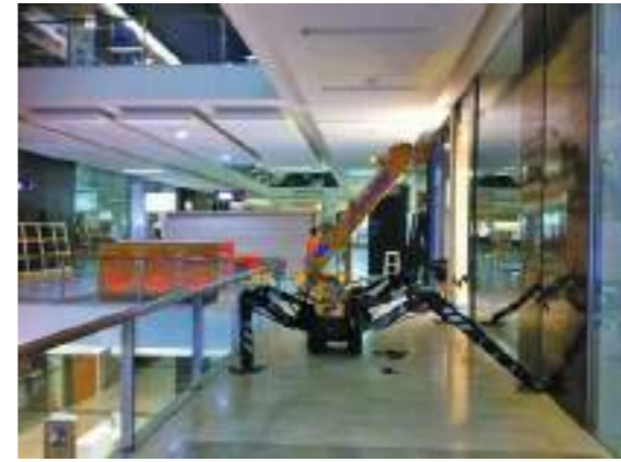
MC285C Glazing at Mall Australia
