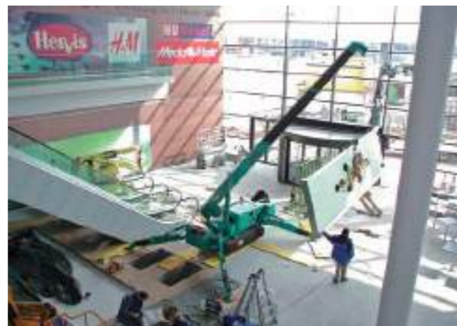
MC305C Panel Installation Mall
