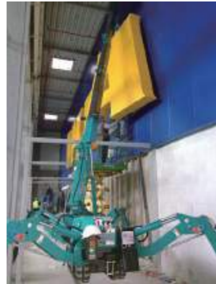
MC285C Sign Installation
