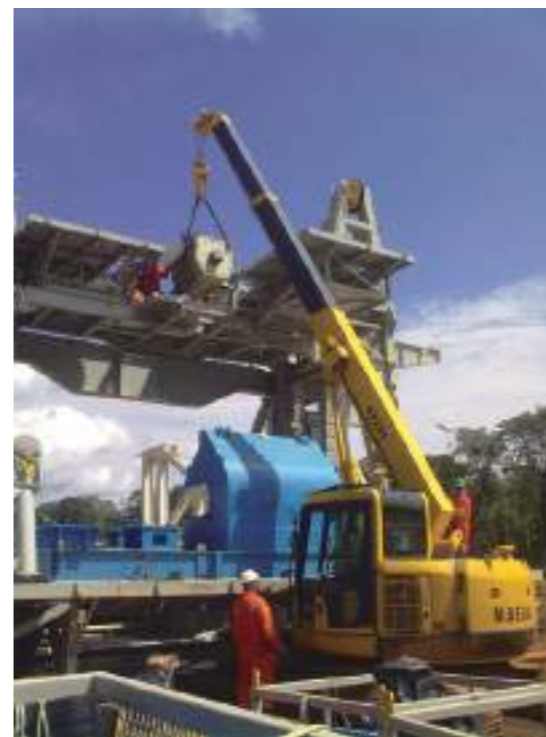
LC1385 Oil Site Rig Up Brazil
