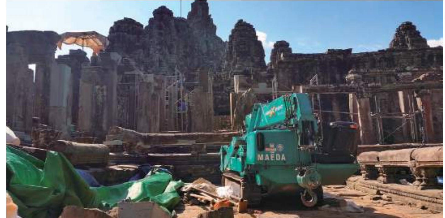
MC305C Angor Thom Restoration
