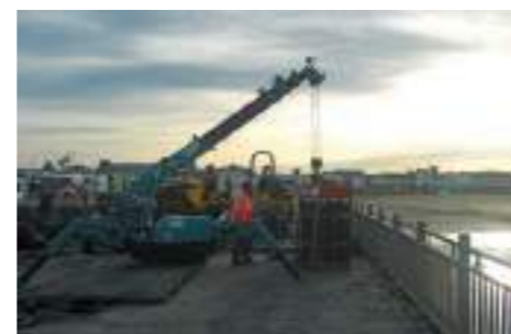
MC285C Weston Pier
